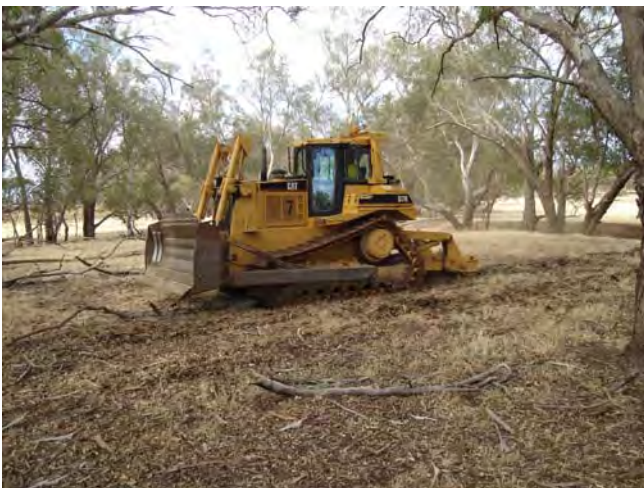
Above: Ripping prior to planting.
